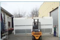
With the transport of the kits, consider the large width and the necessary safety margins. It is absolutely necessary to use an assistant to give directions.
